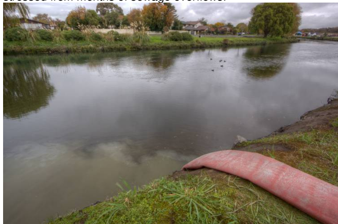
Raw sewage being pumped into the Avon River
