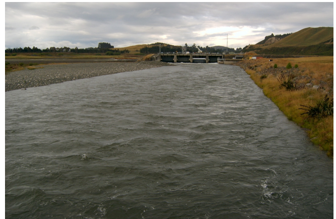
Manapouri Lake Control
