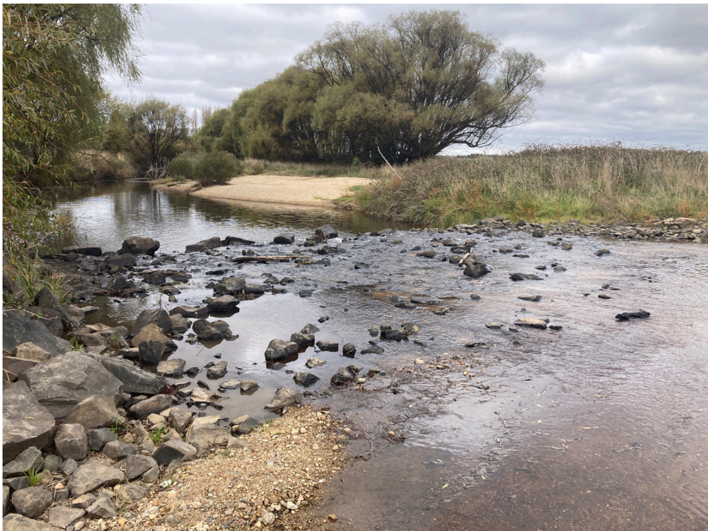
Photo 4: A leaky weir placed along Mulloon Creek.
