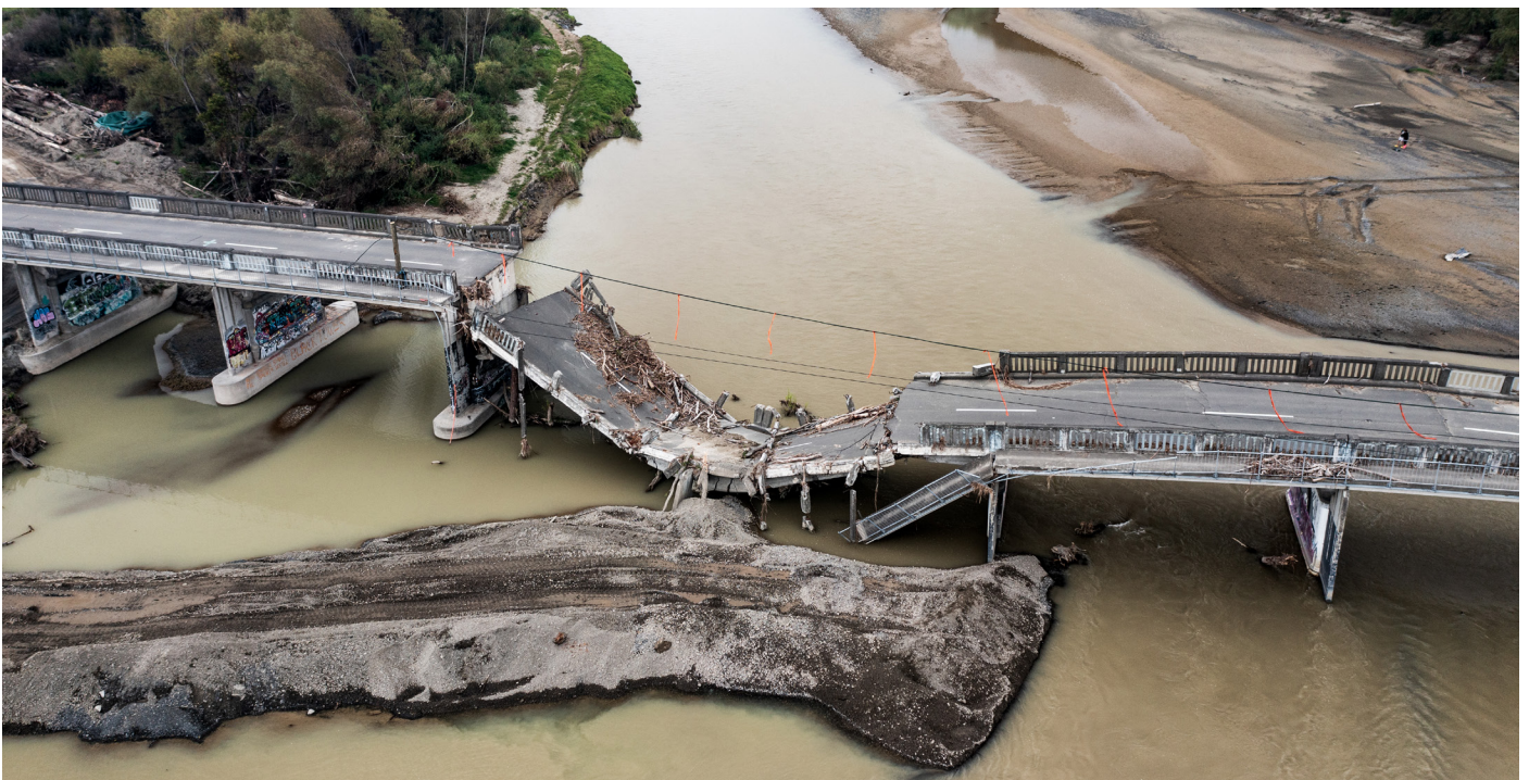
Figure 2: Redclyffe bridge in Hawke's Bay post Cyclone Gabrielle 16/04/23 (Credit: Thomas Kay).
