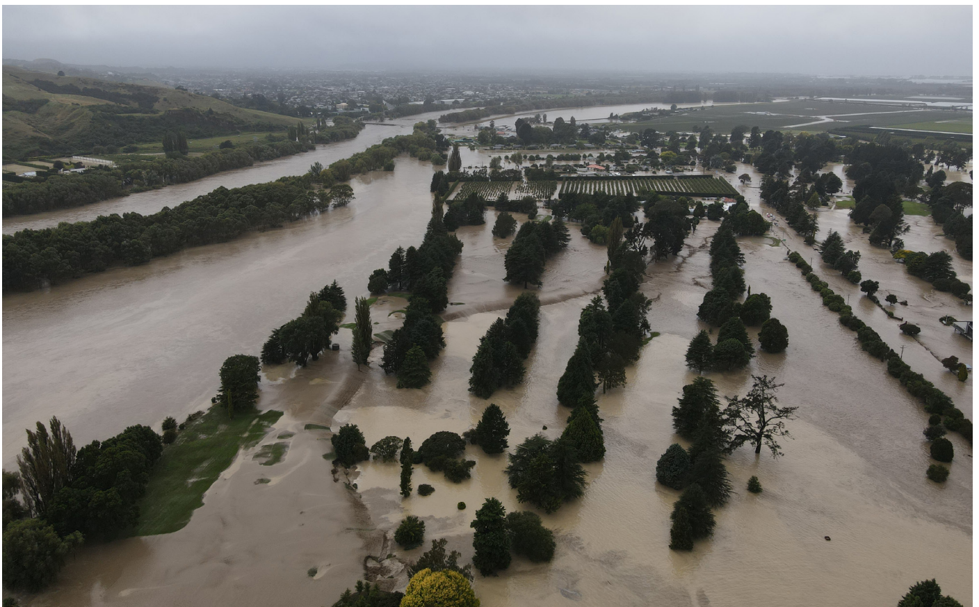
Figure 1: Cyclone Gabrielle flooding from corner SH50 Omarunui Rd in Hawke's Bay on 14/02/23 (Credit: Steve Dighton).
