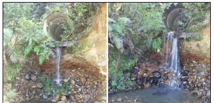
Field installation of fish passage ropes ≈
