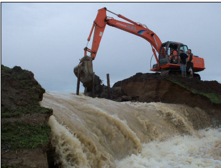
A digger begins repair on a breached stopbank
