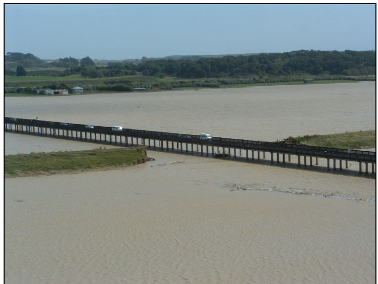
A failed stopbank in Manawatu
