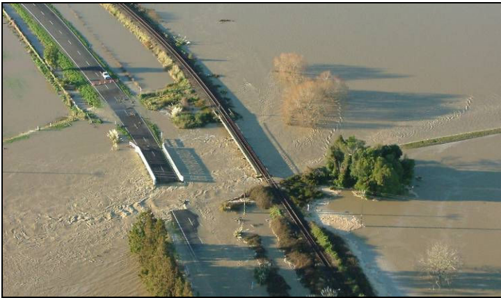
Flooded road and rail bridges in the Bay of Plenty
