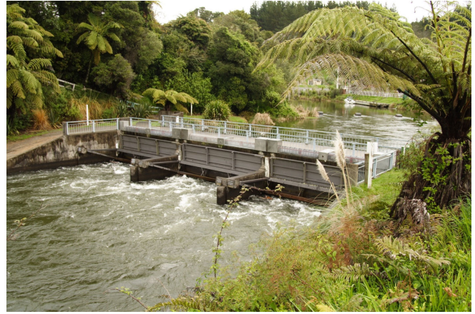
Figure 1: Photograph of Downstream Side of Okere Control Gates Structure from Left Bank of Okere Channel
