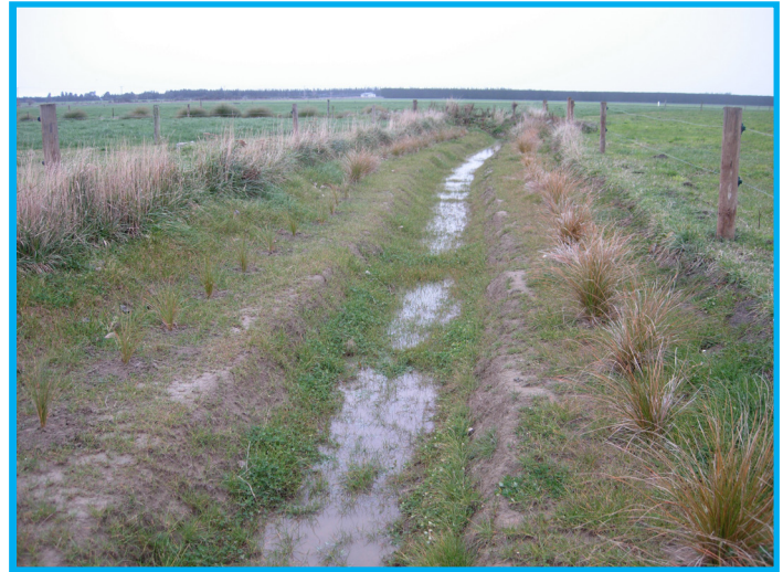
Photo 3: Two-stage channel in June 2016 after grasses and plants have grown.
