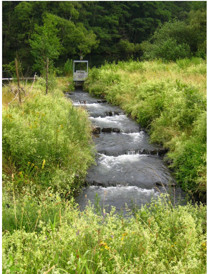
Pool & Boulder-type Bypass Channel, Möhnebogen, Möhne River, Germany
