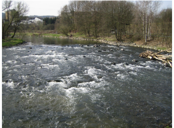
Rock Ramp Neheim-Hüsten, Ruhr River, Germany (Slope = 1:35) in Mean Flow Conditions
