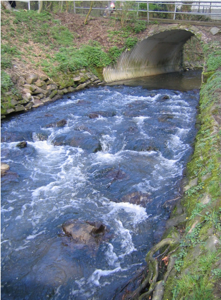
Retrofitted Rock Ramp Below a Perched Culvert, Düssel River, Germany
