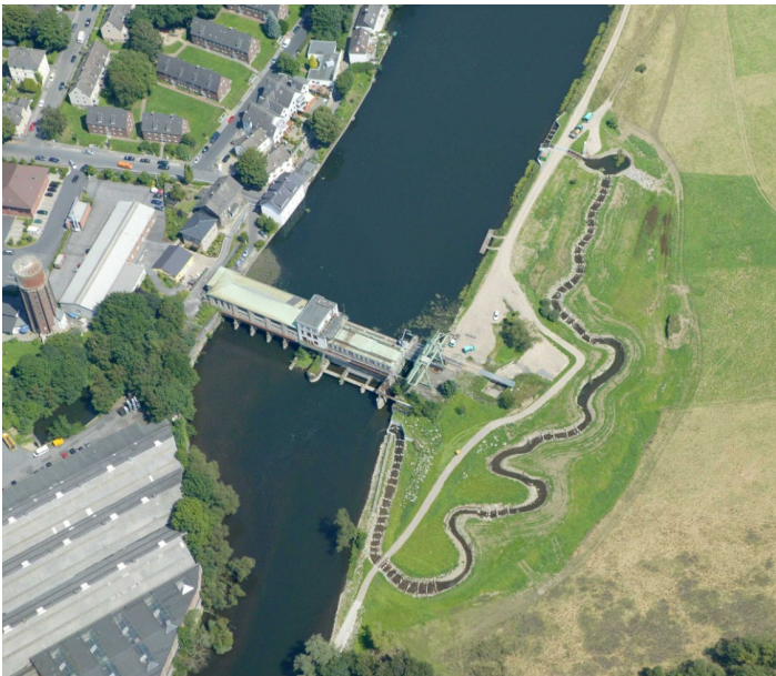
Harkortsee Bypass Channel, Ruhr River, Germany (photo: Ruhrverband)
