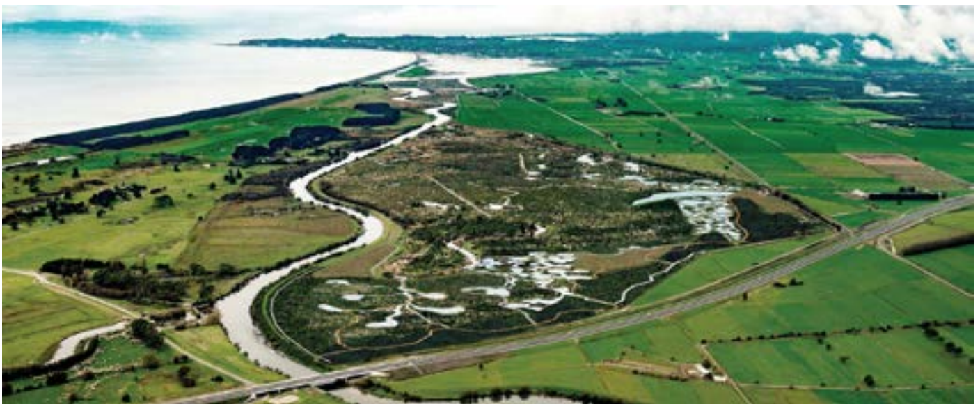
Project area after wetland restoration
