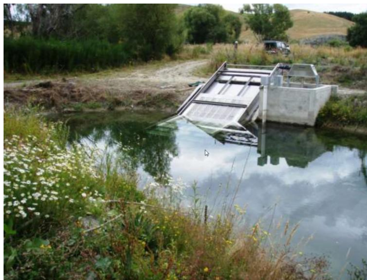
Water intake set up looking across to the Andar screen sketched above
