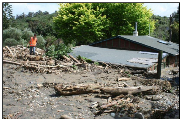
Debris Flow Deposit surrounding property at 64 Pohara Valley Road (2011 – TDC photo)
