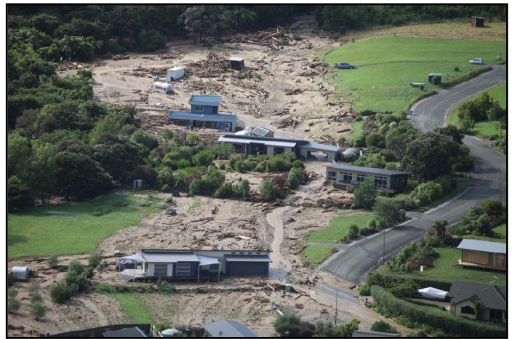
Debris Flow on upper part of Nyhane Drive Fan (2011 - Courtesy of Tim Cuff)
