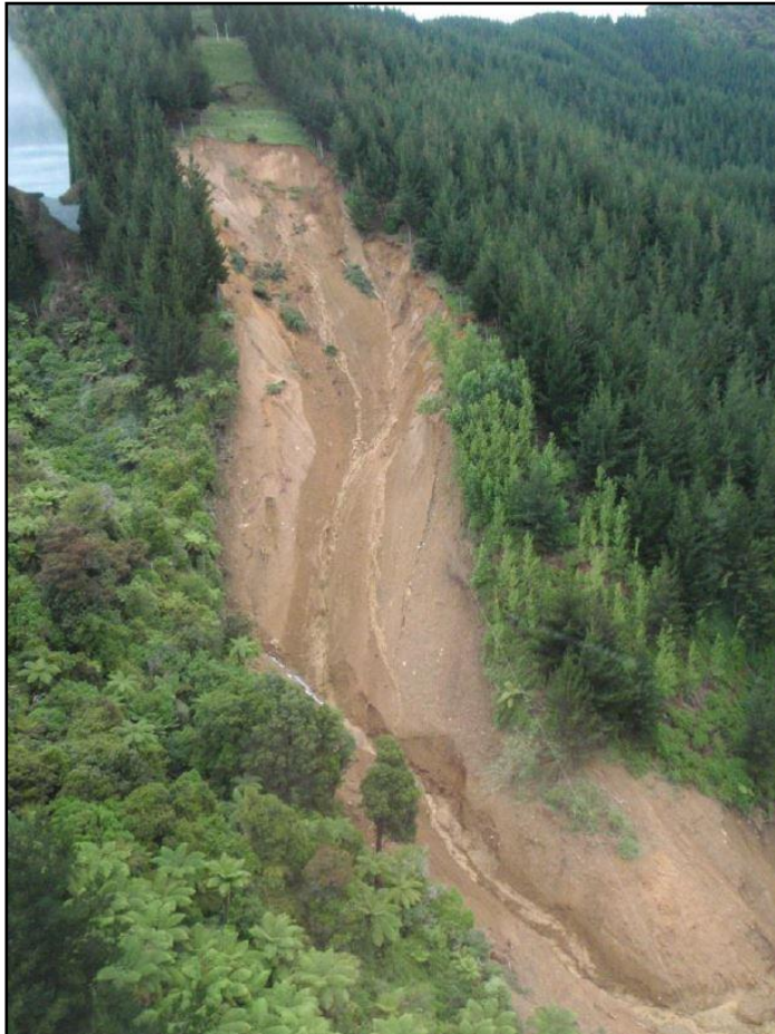
Large Slip in Ellis Creek Catchment (2011 - Courtesy of Paul Woperies)
