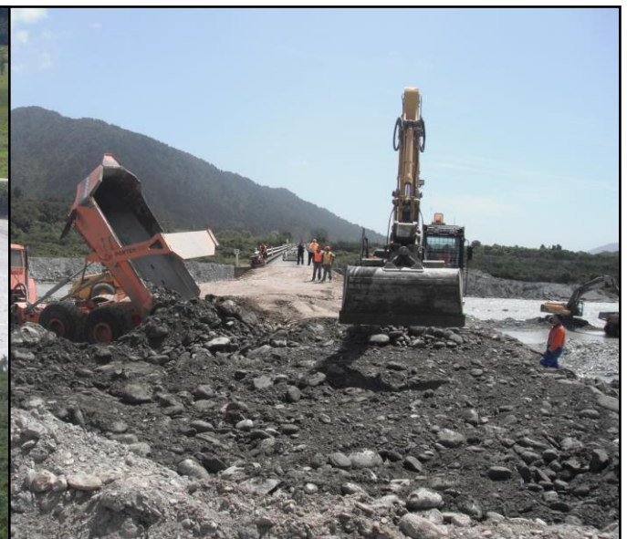
Reinstating the true-right abutment of the Wanganui Bridge following the January 2013 washout
