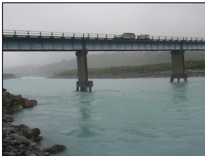
Wanganui Bridge piers in December 2008 looking upstream prior to pier-underpinning works
