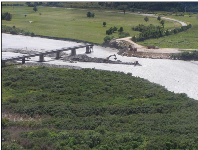
Reinstating the true-right abutment of the Wanganui Bridge following the January 2013 washout
