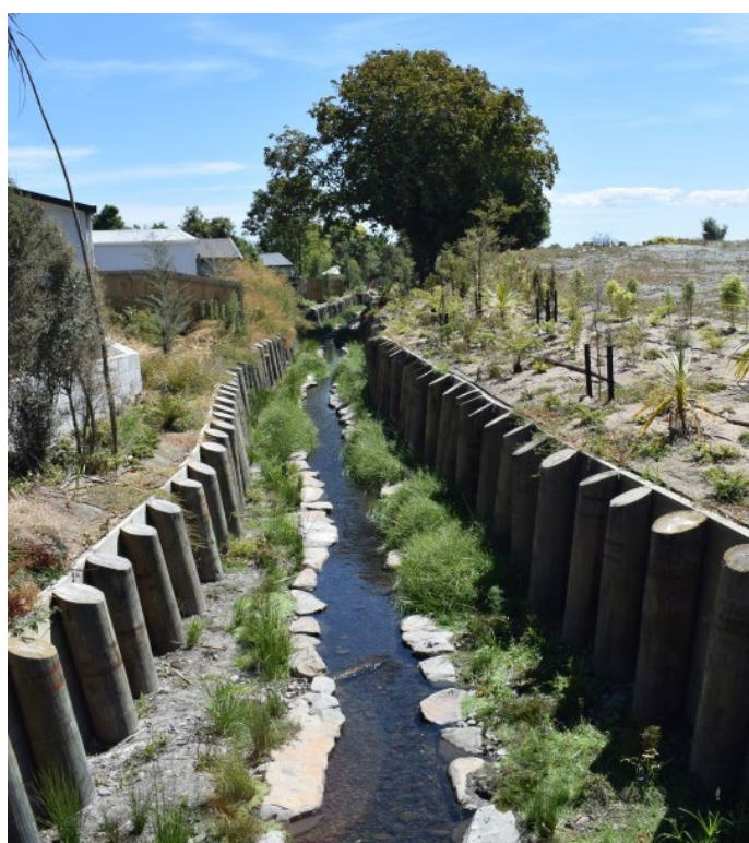
Figure 1: Example of flood remediation work in the Dudley Creek area
