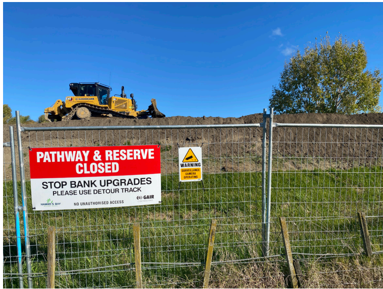
Figure 2. Upgrading flood protection infrastructure, Tūtaekuri River, Hawke's Bay. By Caroline Wood.
