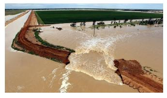
Properties protected by stopbanks (levees) constructed and maintained to reliably withstand a design flood with a frequency of 0.2% Annual Exceedance Probability (AEP) including a minimum 0.9 m freeboard are considered to be in a reduced hazard area. While terminology and appetite for accepting risk varies from one insurance company to another, a majority of insurance companies are interested in understanding the risk associated with the 1% AEP and 0.2% AEP floods.
